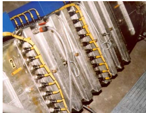
Figure 1a (top) UV-disinfection plants in water work Pitkääkoski/Helsinki, Finland. Figure 1b (bottom) several plant sensors can be seen at the side of the UV-plant.
