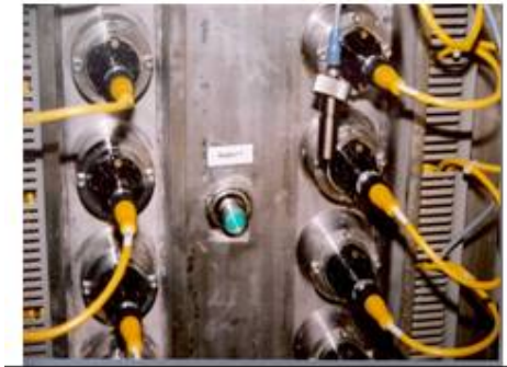
Figure 1a (Top) UV-disinfection plant for 1 800 m 3 /h in Vienna. Figure 1b (Bottom) sensor and sensor port.
